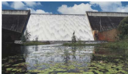
(Tinaroo Spillway. Photo Courtesy Sunwater)
